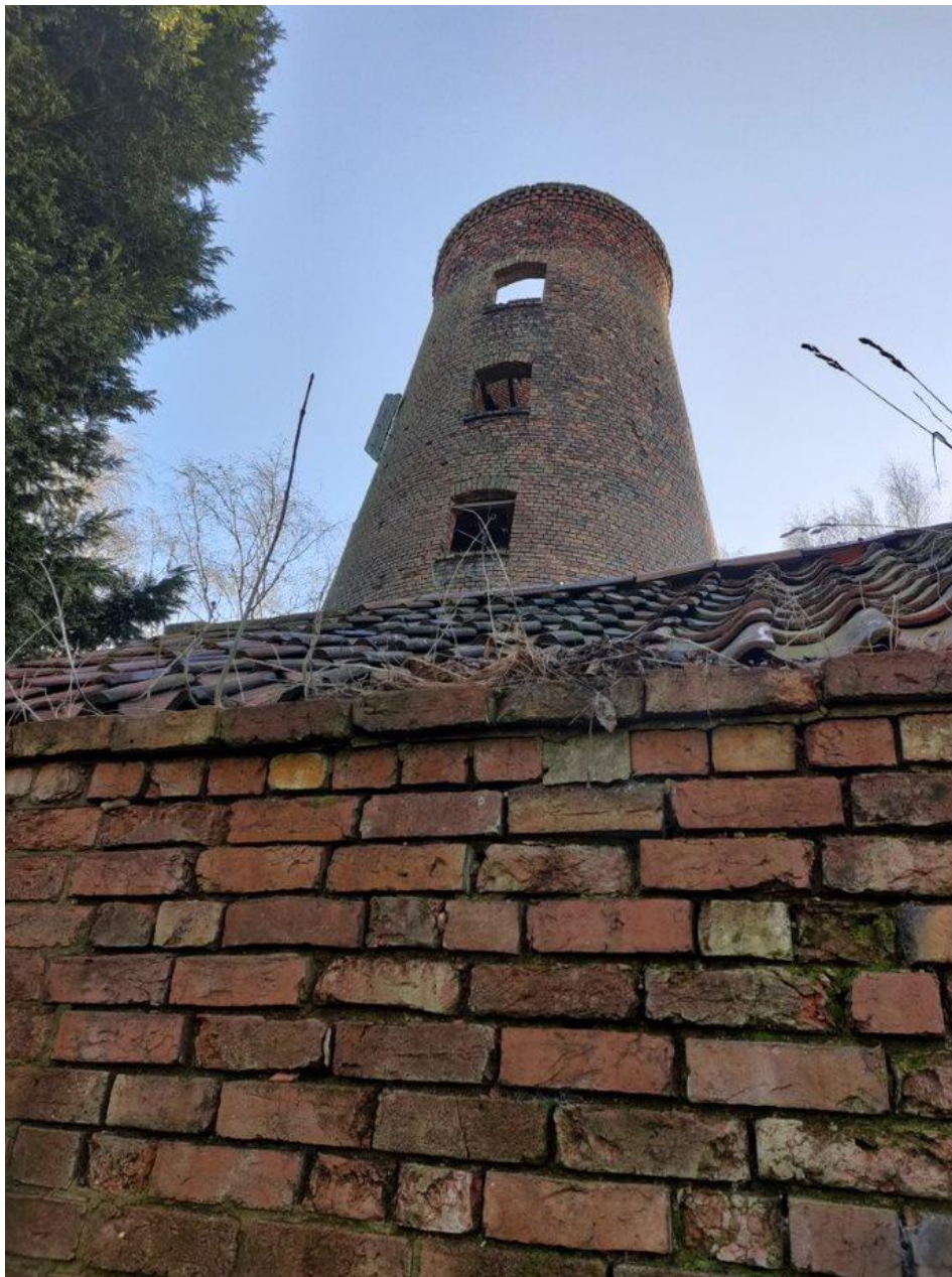
Source: Mott MacDonald (2023)
